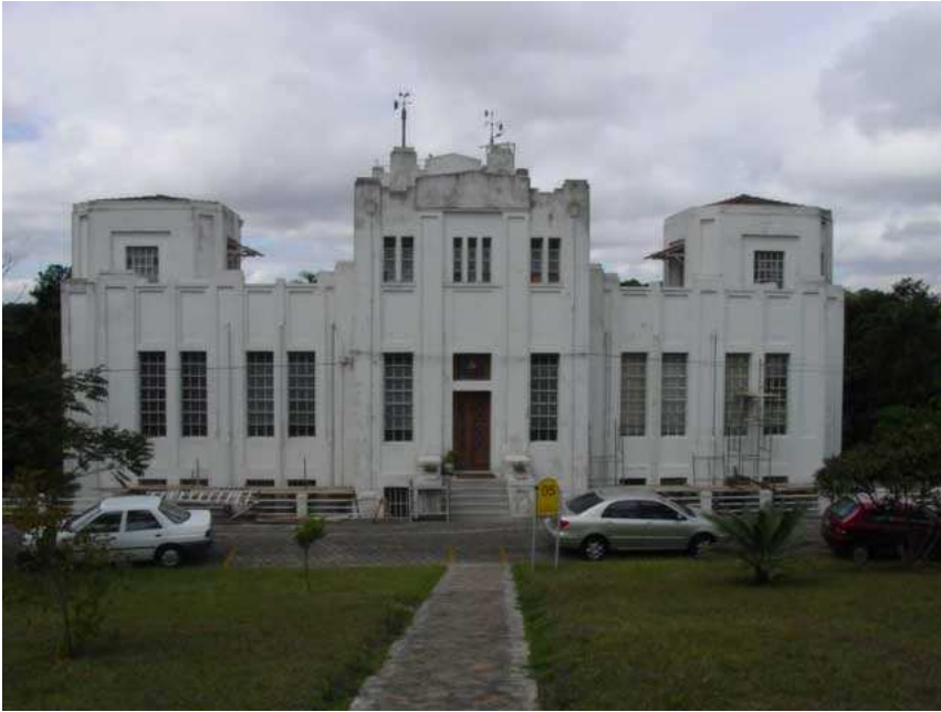
Figure 4. Instituto Astronômico e Geofísico (IAG/USP), building from 1932. The site is now a state outreach science Park and the IAG/USP staff was relocated at the University of São Paulo main campus. (Courtesy IAG/USP)
