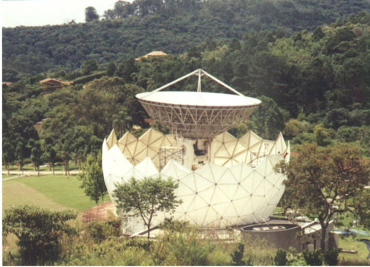
The Itapetinga 14m telescope during the change of radome
