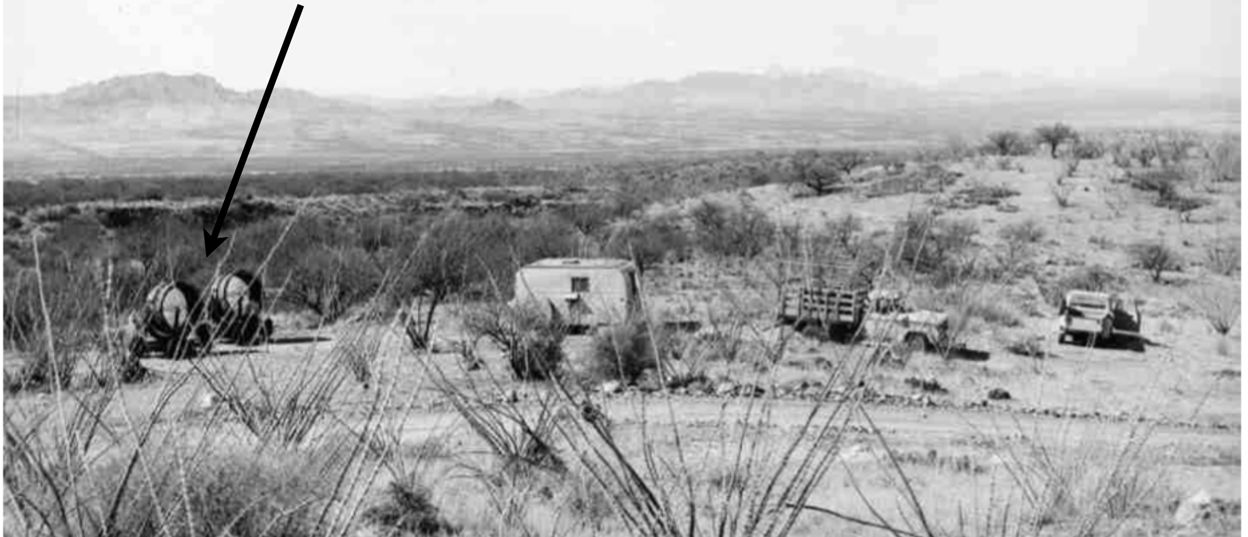
FIGURE 1. The first TeV gamma-ray observatory in the United States consisted of two 1.5m telescopes (made from World War II searchlight reflectors) above (left center); the telescopes were manually operated and were located at a dark site in southern Arizona during the winter of 1967-8 [10]. The telescopes were directed (by eye) at a point ahead of the position of the putative source so that the earth's rotation swept the source through the field of view. Power came from an electric generator on the back of the truck (center right) and the pulse counting electronics were housed in a small trailer (center). The system was mercifully free of computers and the analysis was done offline with a mechanical calculator. No sources were detected.
