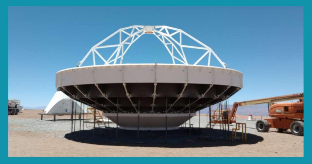
The LLAMA reflector, constructed by VERTEX, was in the process of been mounted by INVAP, on the site of the observatory, in Alto Chorrillos, when the order to stop the work came. Since then the reflector is precisely at the same place, with no protection.
